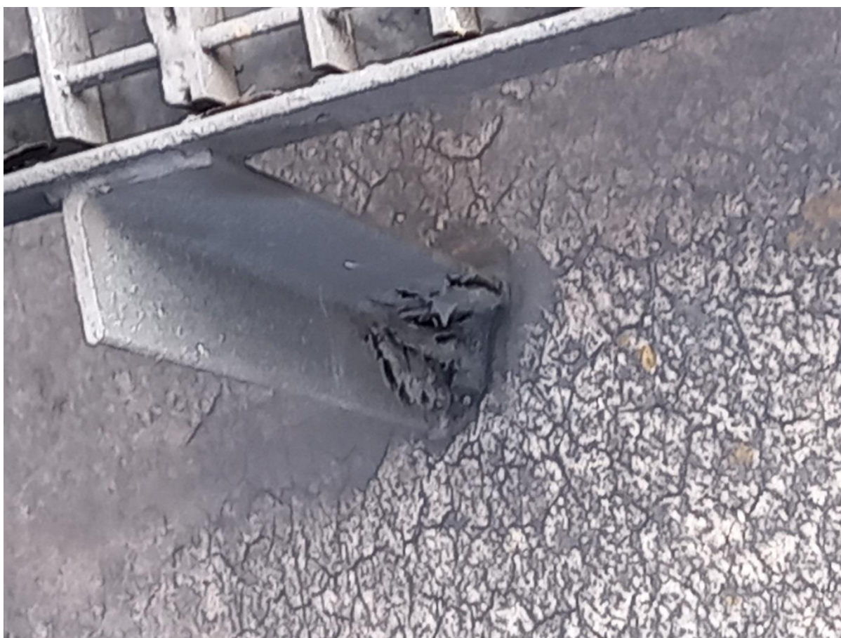
Photo of a rusted support on the Tank for the landing platform
