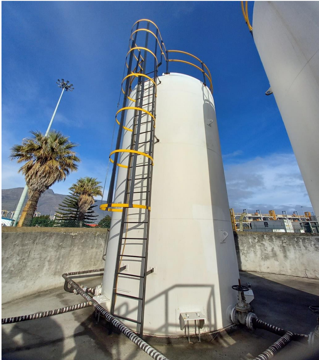
2 x 39000 L Tank: Diameter 2.82 m x 6 m Long
