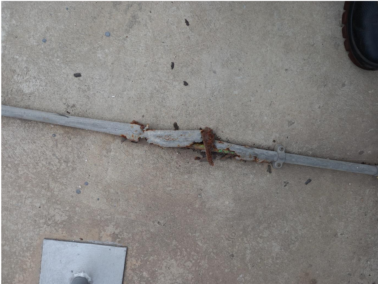
Earthing cable cover is broken and in a poor condition
