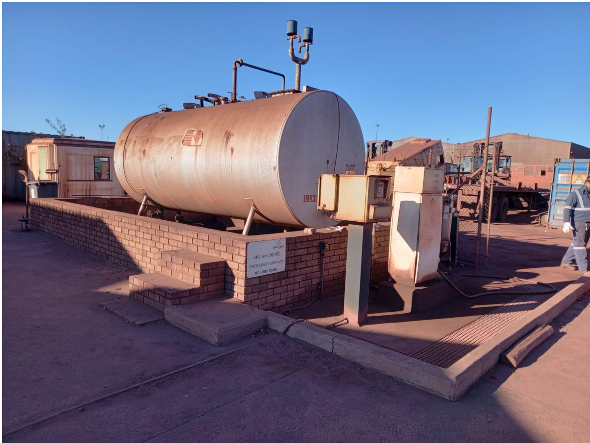
23 000 L Tank: Diameter 2.3 m x 5.4 m Long Bund-wall
