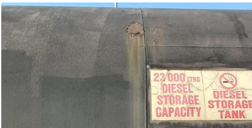
Photo of a corrosion on the Tank
