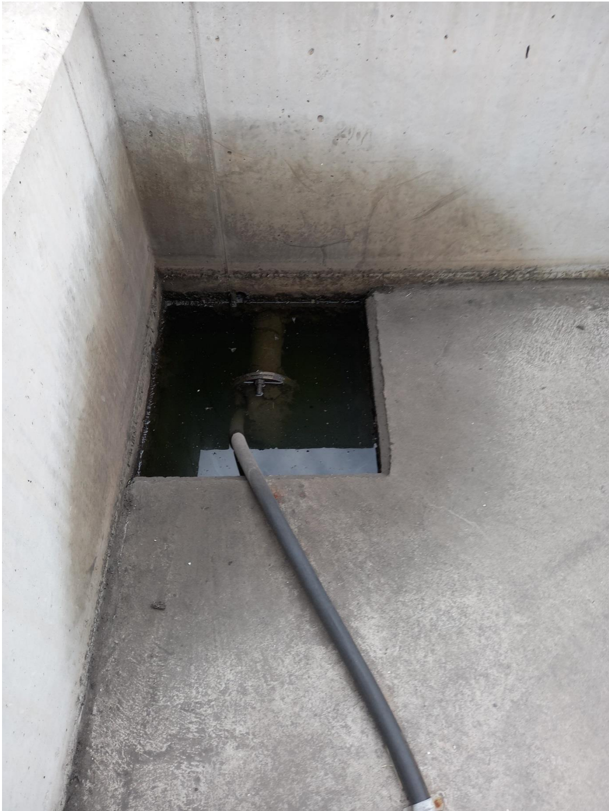
Strom water drain is choked
