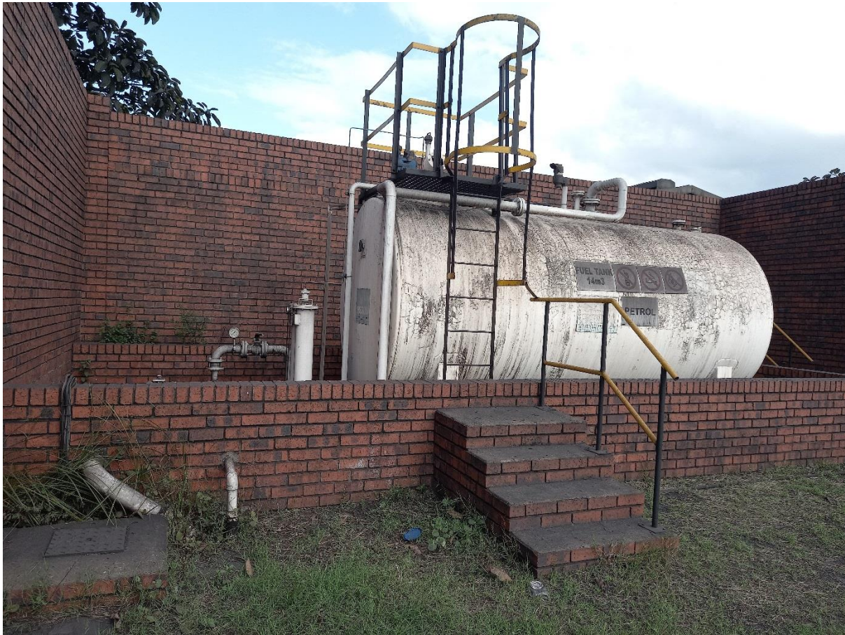
Photo of a Petrol Tank to be demolished along with piping and the bund area
