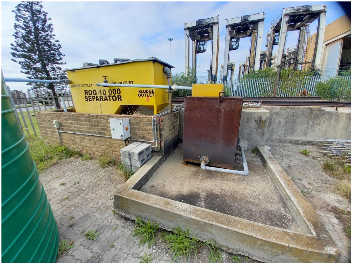
Oil spillage collection and filter area
