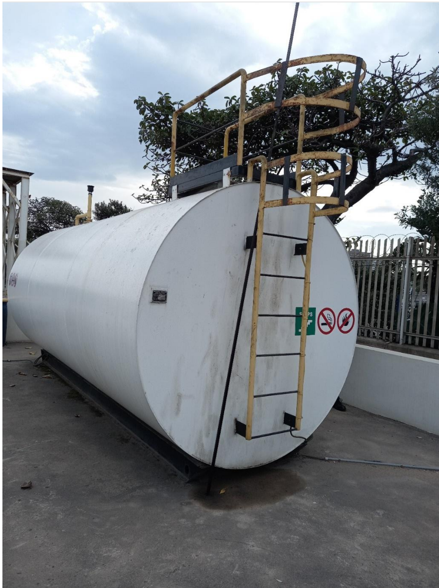
Platform, ladder etc. are rusted
