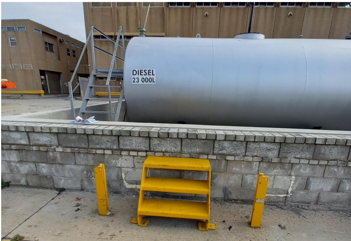
Small size and short steps with no handrails
