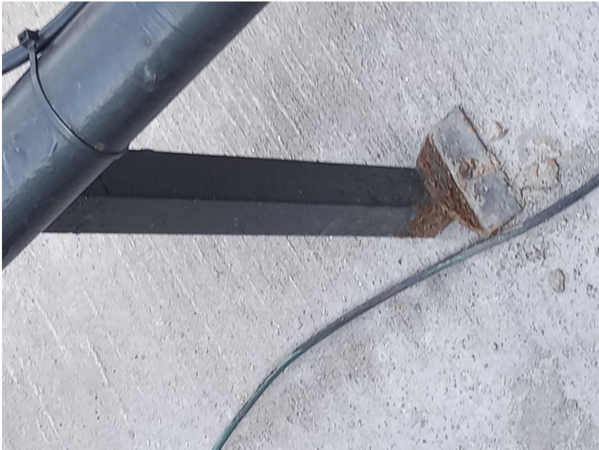
Piping supports needs to be replaced
